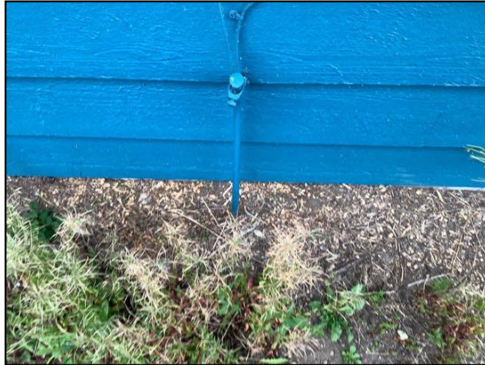
21. Copper - ground rods
