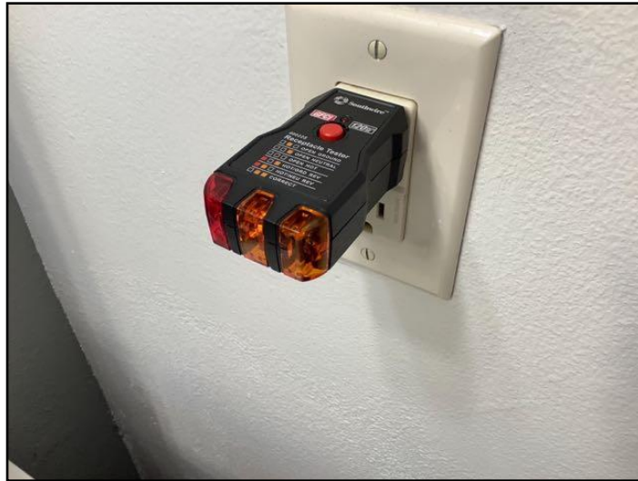
32. Ungrounded GFCI in Bathroom
