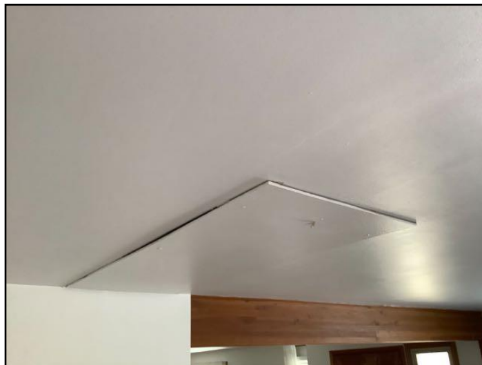
42. Inadequate insulation
