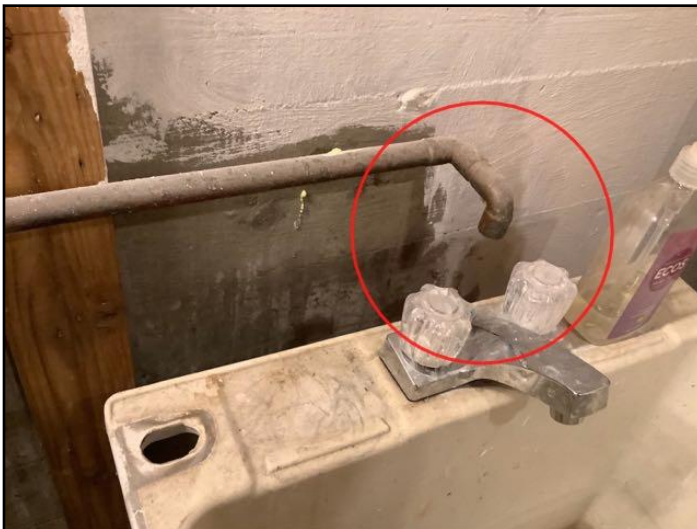
50. Discharge arrangement poor
