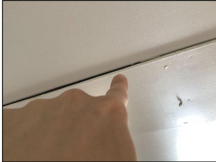
43. Inadequate weatherstripping
