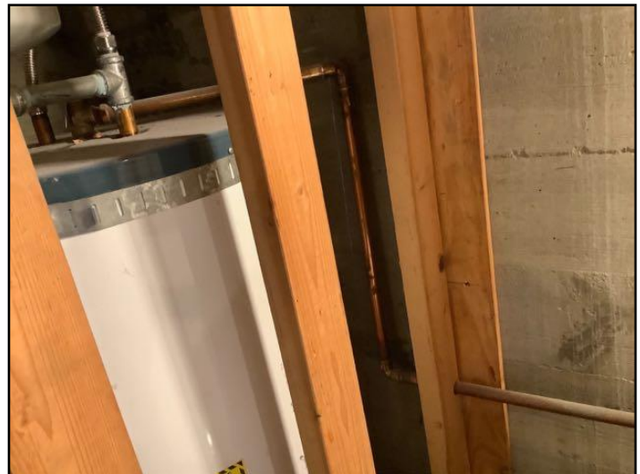
51. Discharge arrangement poor
