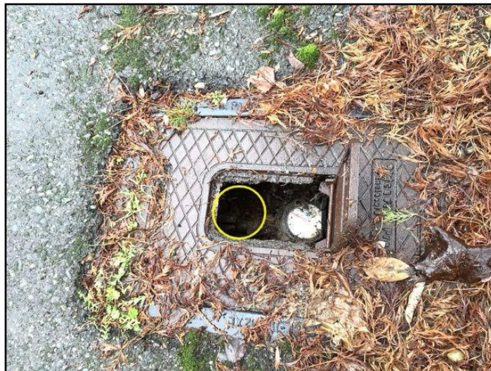
45. Water shut off at the Meter
